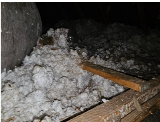
2612-5 Insulation Typical Interior
