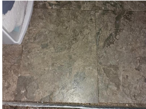
2612-4 12"x12" Floor Tile/Adhesive Typical Interior Bathrooms
