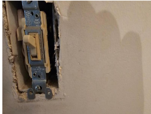
2612-2 Drywall/Joint Compound Typical Interior Walls/Ceilings
